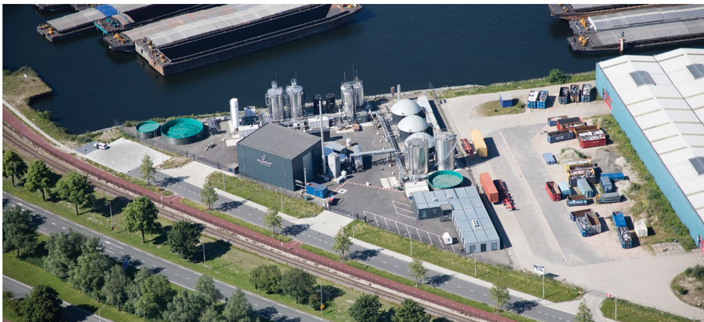
An aerial view of ChainCraft's demonstration facility at the Port of Amsterdam. Photo courtesy of ChainCraft.
